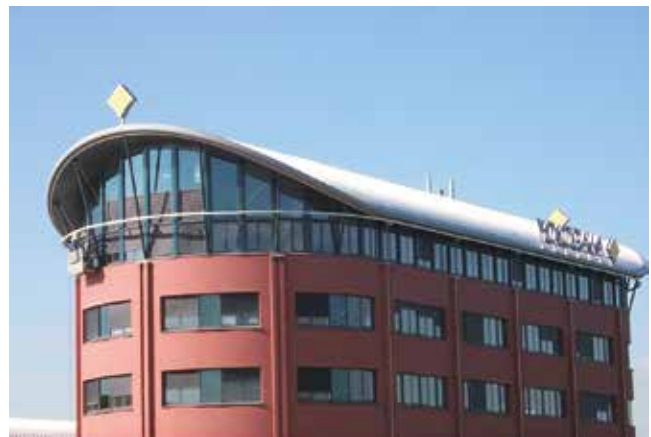
Curved installation for window cleaning equipment
